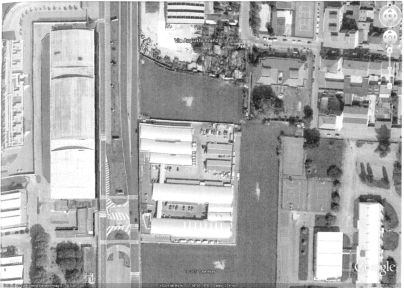
Vista aerea aree denominate "A"- "B"
