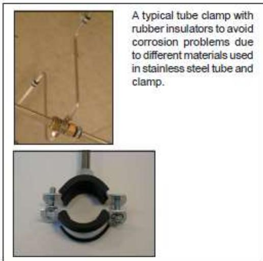
A typical tube clamp with rubber insulators to avoid corrosion problems due to different materials used in stainless steel tube and clamp.
