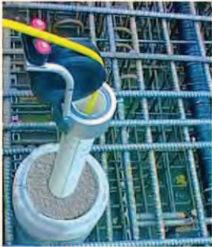
Pulley and cable stop
